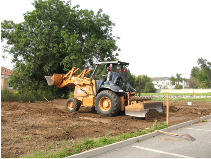
Grading in Progress
