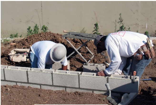
Retaining Walls Were Built
